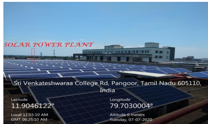
SOLAR POWER PLANT
